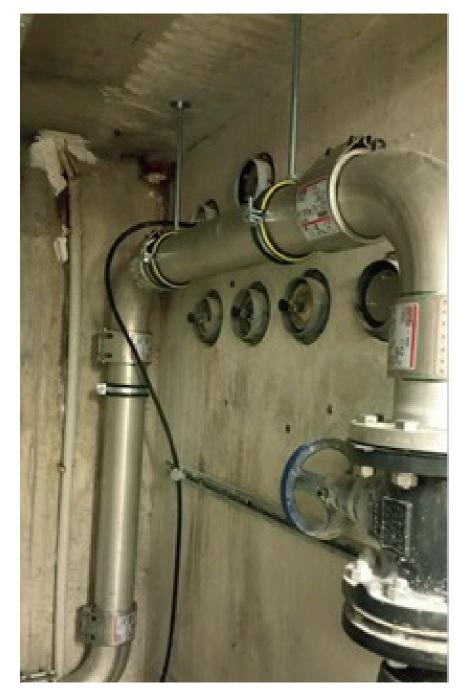
The quick, easy and reliable Straub mechanical joint is an alternative to welding or flange connections.
