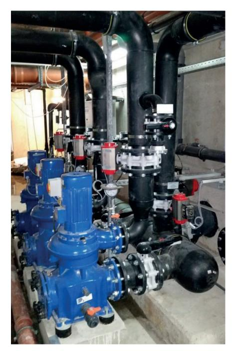
Our piping system made of polyethylene is used since decades in areas of application where the pipe system has to meet high standards of durability and reliability.
